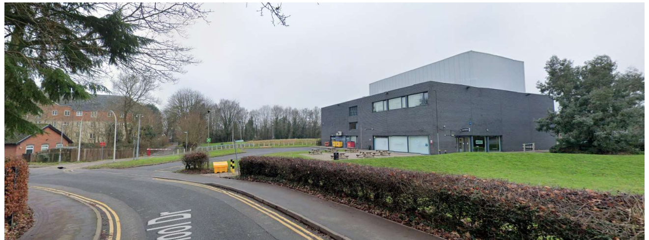
Photo from google street view looking north towards the School Drive access to the Artrix Centre
